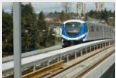
Rail signalling systems
